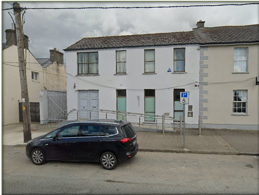
Figure 5 – Existing Front of Building (© Google)
